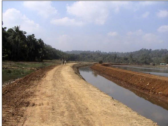
Fig- 8.1 Saline reclamation bund and drainage training works at Chouldari, These works are beneficial for land resources preservation and stopping salinity ingress in the subsurface, S.Andaman.
