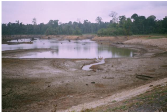
Fig-5.2.4.10 State of R.K.Pur Dam, Little Andaman after 26.12.04 Earth Quake
